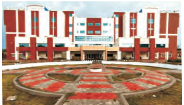
Upgradation of Medical College institution under PMSSY Phase - III Hospital PMCH, Dhanbad
